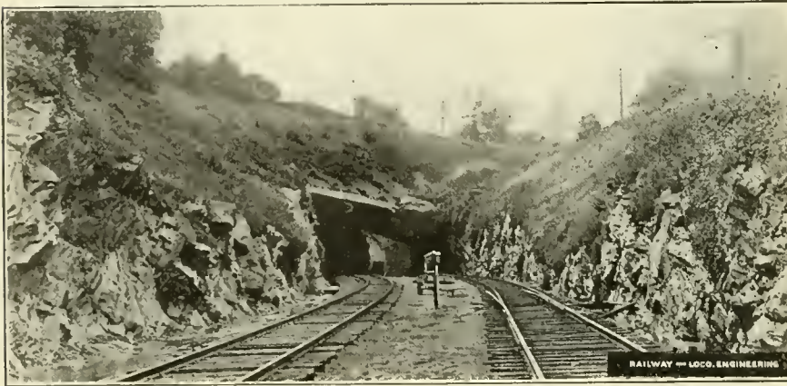
MANUNCACHUNK TUNNEL ON THE LACKAWANNA SHOWING DERAILING SWITCH NEAR ENTRANCE.
